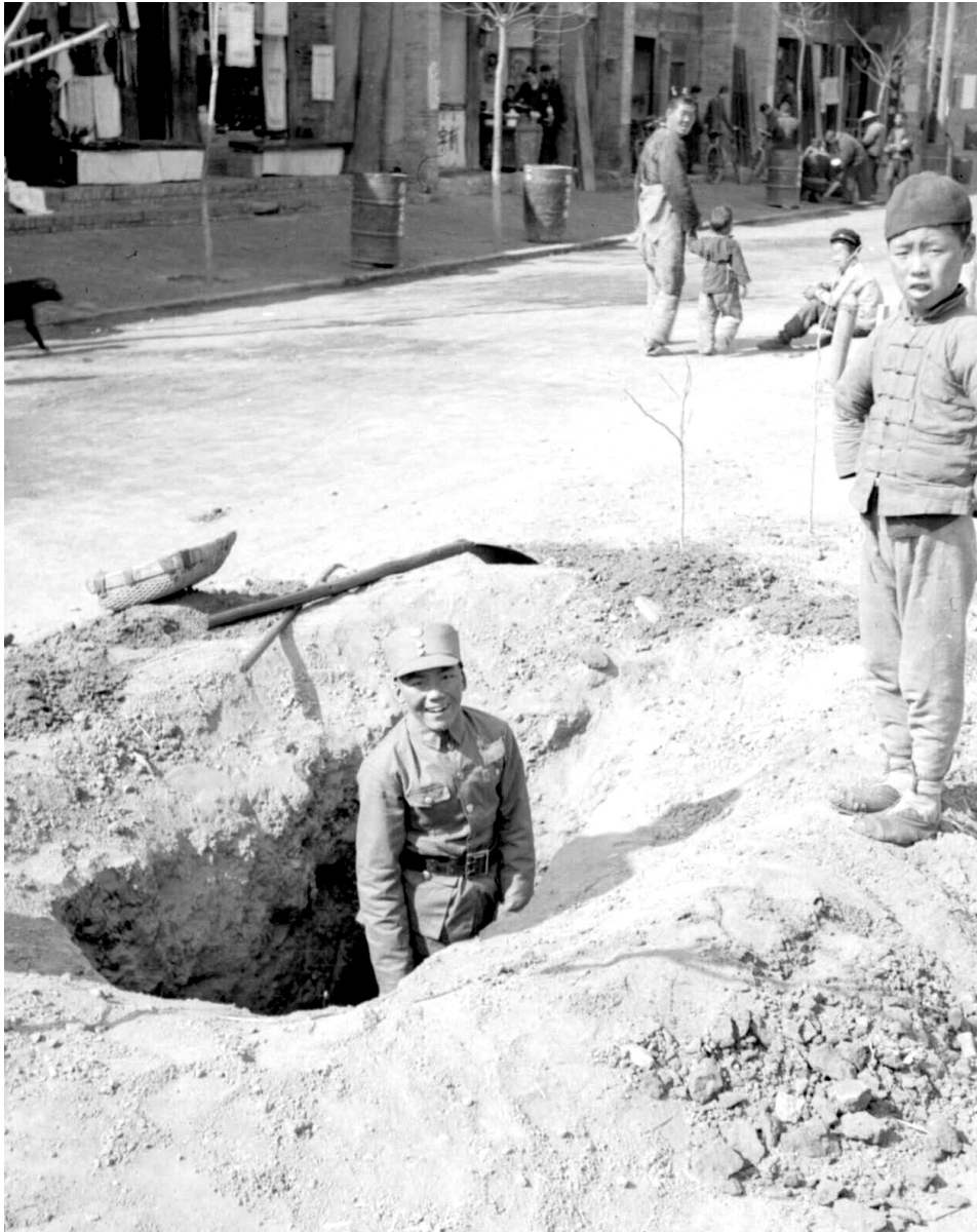
Figure 5.8: Digging a bomb shelter in Cheng-Chou [ ZhengZhou ]. Here, because of the high water table, only shallow shelters could be dug.
