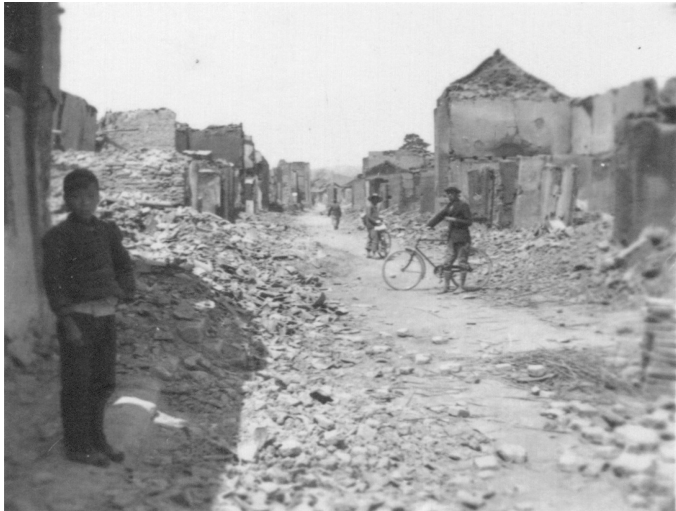
Figure 2.15: The destruction at Ku Cheng. (Left) The Christians at Ku Cheng set up food stalls for fleeing refugees. (Right) The burned-out church at Ku Cheng.
