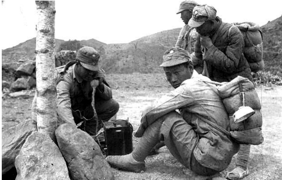
Figure 2.2: Telephone connection in guerrilla territory.
