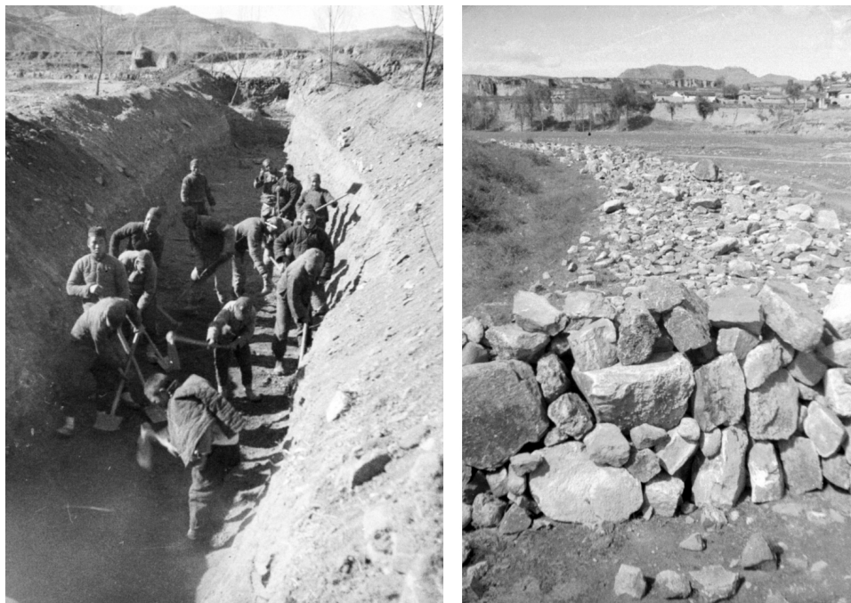
Figure 3.6: (Left) Chinese peasants, under military direction, dig a deep ditch across a river flood plain to stop Japanese mechanized transport. (Right) A road blocked by stone walls and strewn stones.
