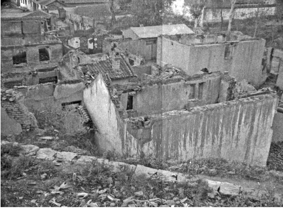
Figure 1.4: Ruins in Qinxian seen from town wall.
